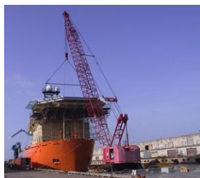
Setting Heli-Deck With 150' Of Boom
